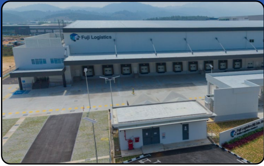
Warehouse At Kulim Hi-Tech Park, Kedah.
