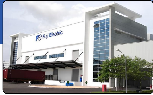
Semiconductor Factory At Kulim Hi-Tech Park, Kedah.
