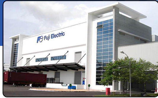
Semiconductor Factory At Kulim Hi-Tech Park, Kedah.
