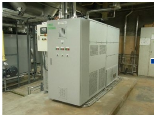
Dimensions: 2,200×1,200×1,760H (Can be carried in via an elevator by splitting the system)
